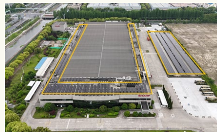
Solar power system
